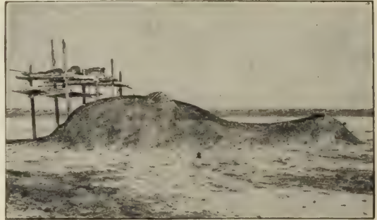
EARTH-COVERED HOUSE, WESTERN ESKIMO. (MURDOCH)
